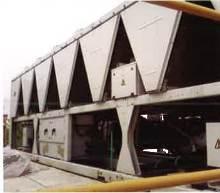
AHU & Chiller(Centralized Air-Conditioning)
