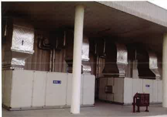
AHU & Chiller(Centralized Air-Conditioning)
